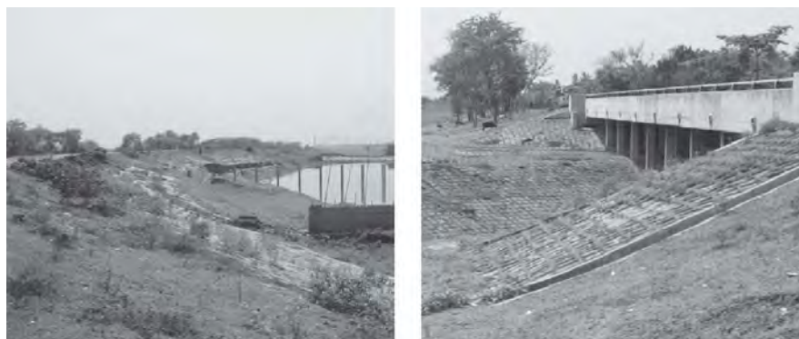
Figure 5-3: Earth embankment along the river (left) with stabilization (right) (ADPC, 2005).
